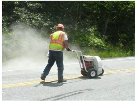
B. Cleaning the crack with a blower.
