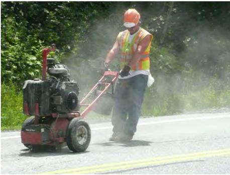
A. Routing the crack.
