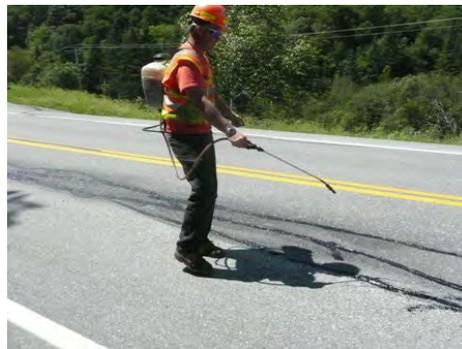
E. Water spraying to cool cracks quicker.
