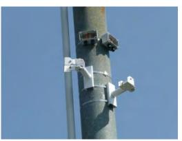
Figure 5: Mounting brackets and electrical boxes.
