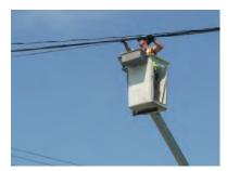
Figure 11: Running the wire across intersection.
