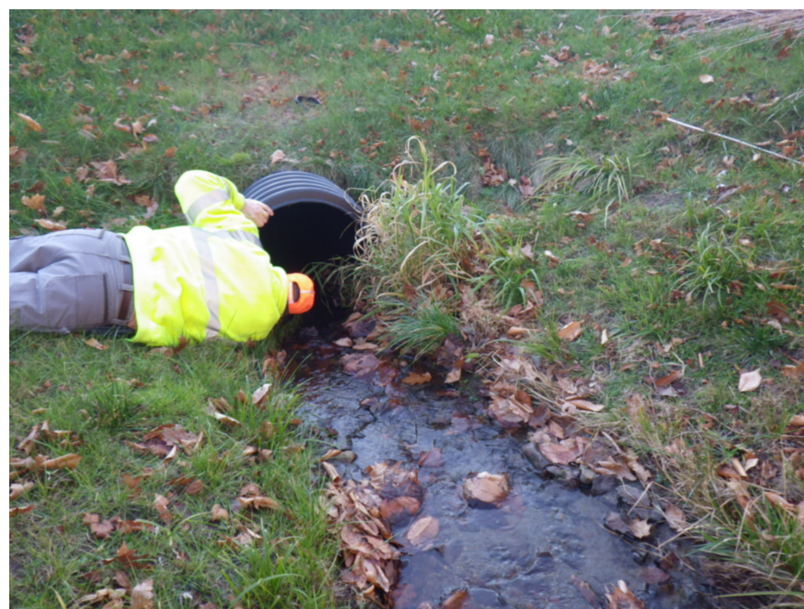
Figure 1. Culvert Inspection Using End of Pipe Method.
