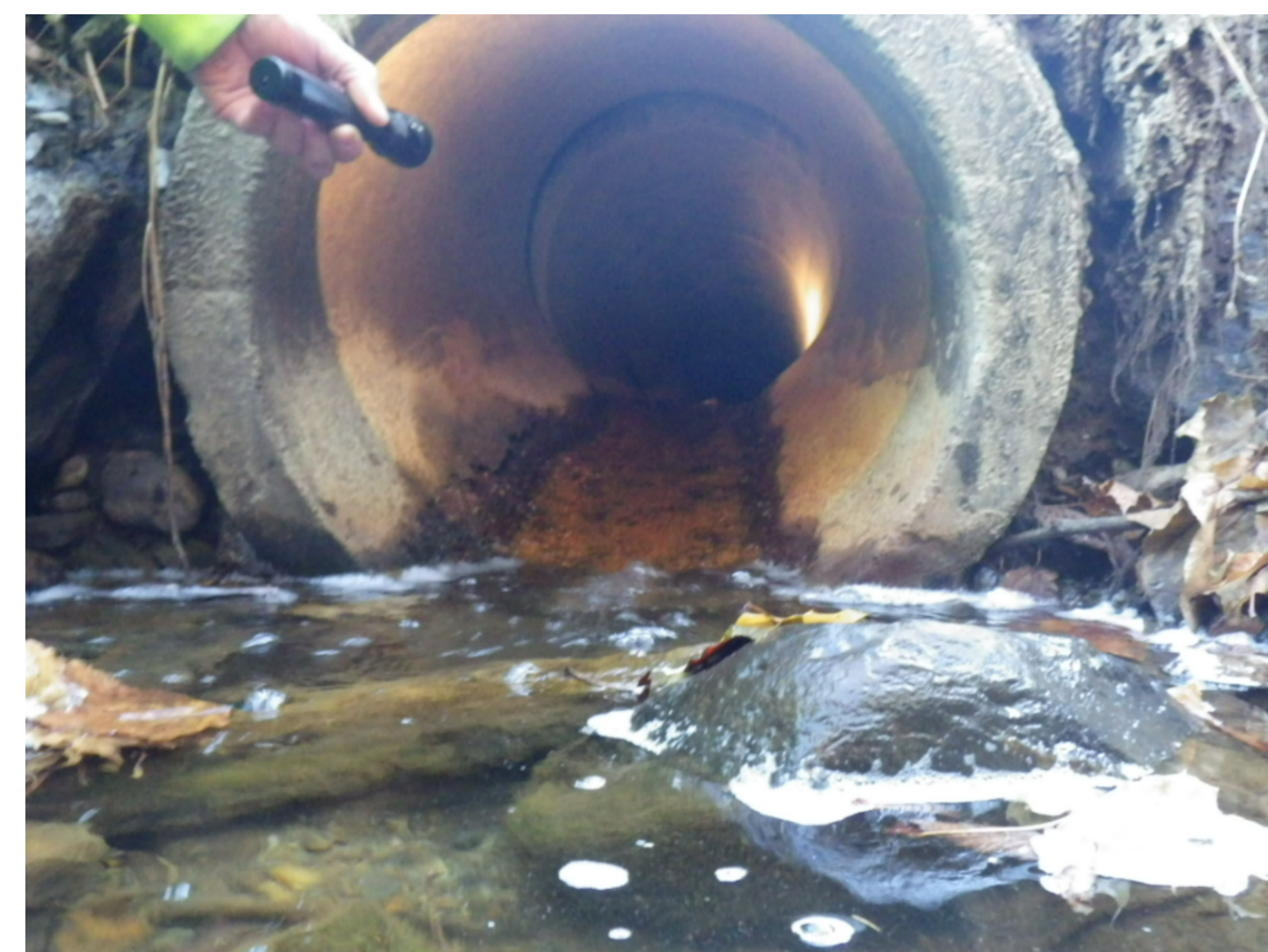
Figure 1. Culvert Inspection Using End of Pipe Method.
