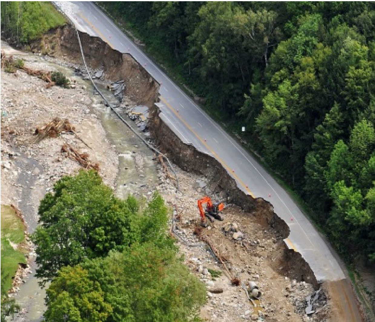
Route 4 failure due to erosion on Mendon Brook during Tropical Storm Irene. Source: L. Grange and Mansfield Heliflight.
