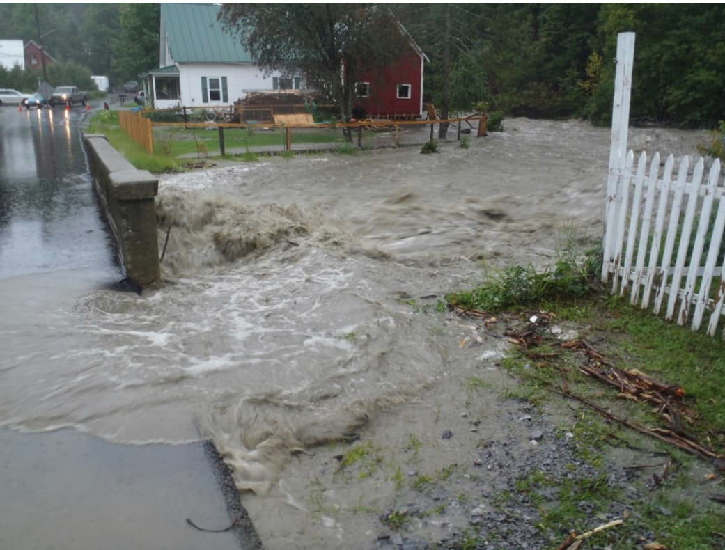
Great Brook Brook Road Overtopping, 50-Year Flood Plainfield, VT 5/26/2011 Photo taken by G. Springston
