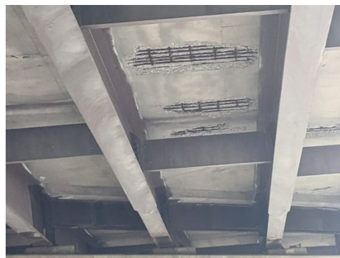
Delaminated bridge deck bottom
