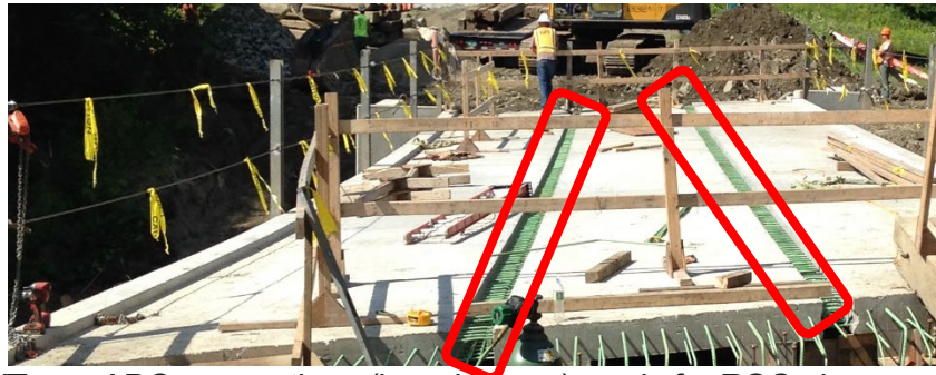
VTrans ABC connections (in red boxes) ready for RSC placement.
