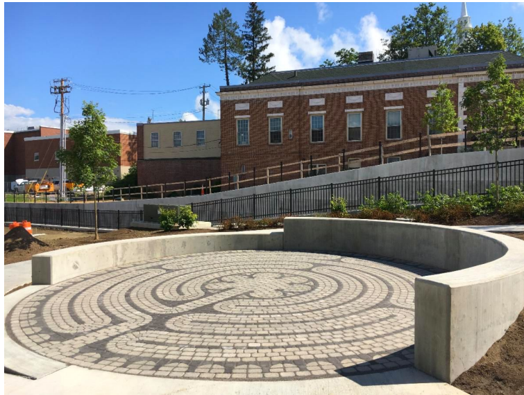
The above photo shows the completed stone paver labyrinth in Lazarus Park.
