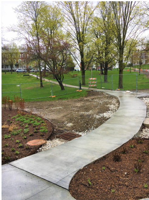
Spring is in the air in Downtown Middlebury! The above photo shows new concrete sidewalks in Triangle Park.
