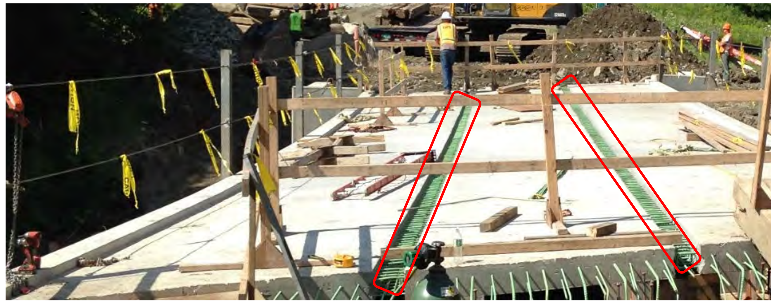
Figure 1. VTrans ABC Connections (in red boxes) ready for RSC placement
