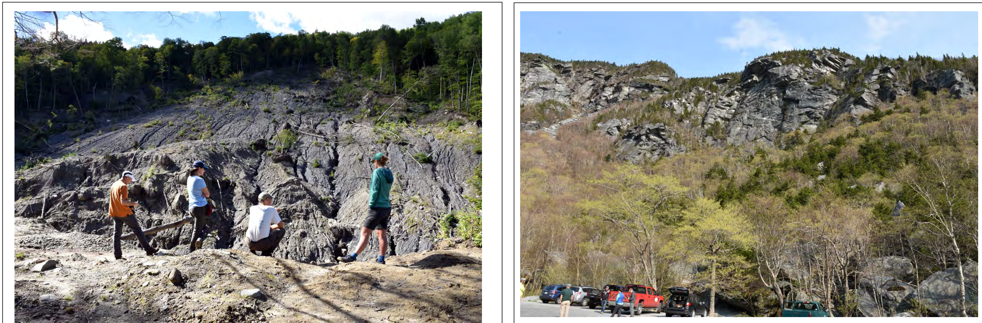
Figure 1. We are conducting annual monitoring surveys of the Cotton Brook landslide (Waterbury- left) and rockslides in Smugglers Notch (Cambridge-right).
