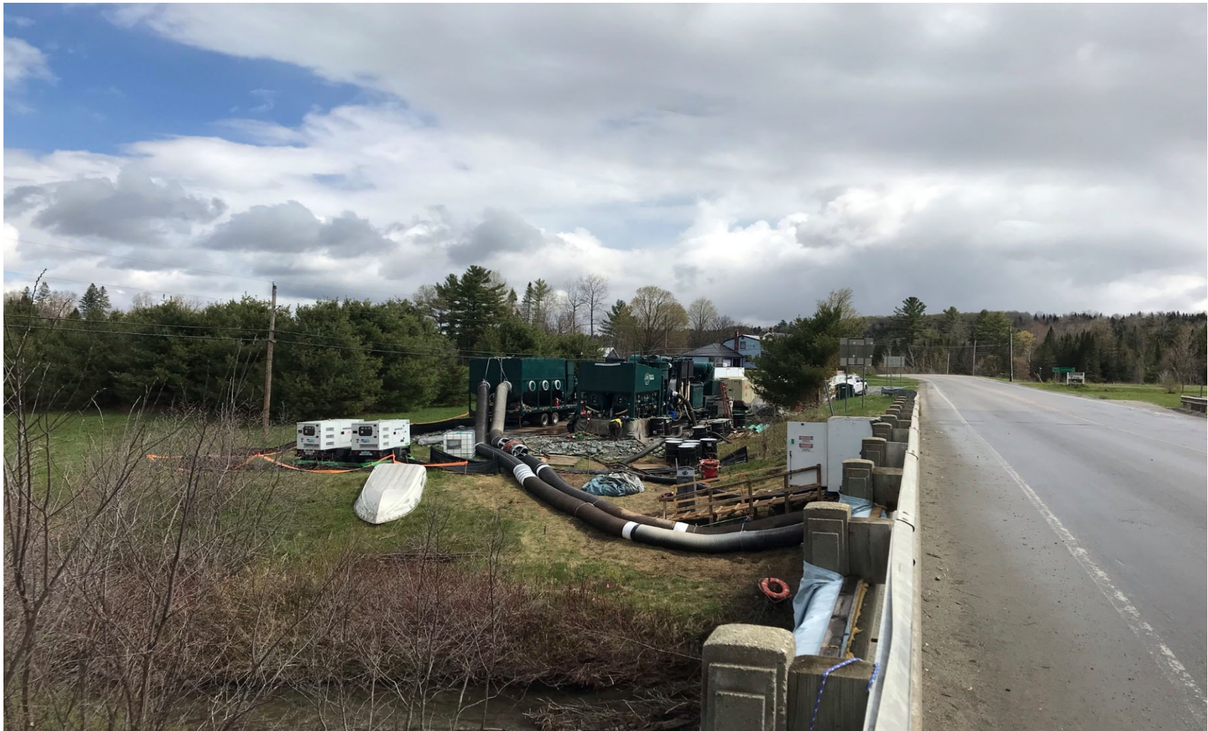
FIELD METALIZING A STEEL BEAM BRIDGE
