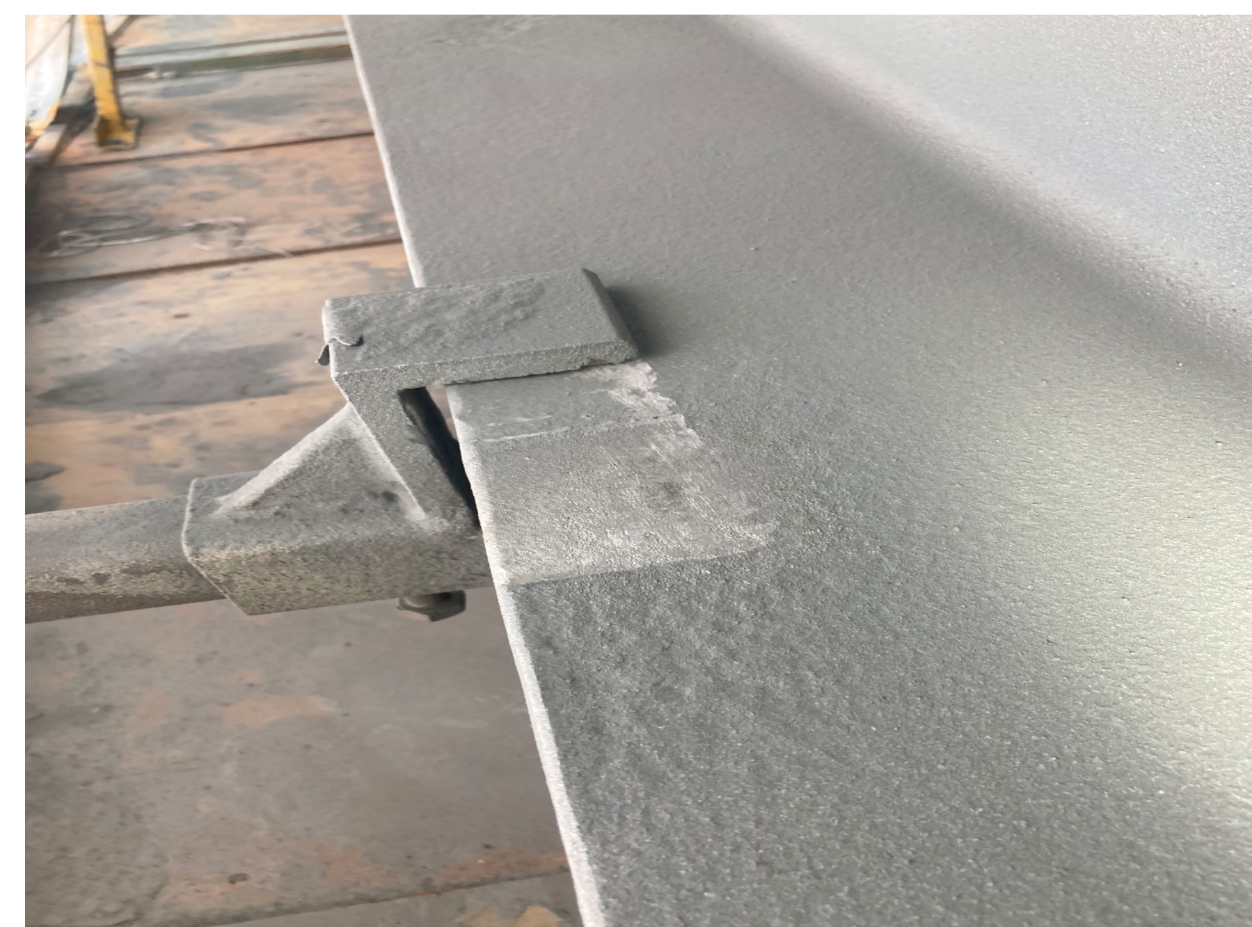
Repairing Staging Hanger Locations
