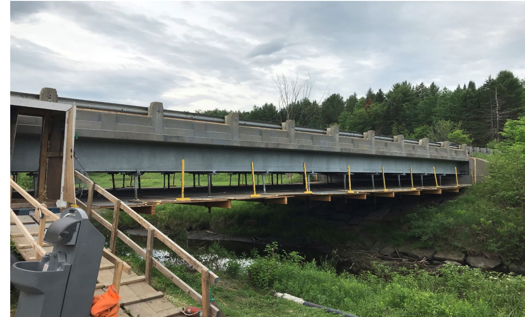
Installation of Staging
