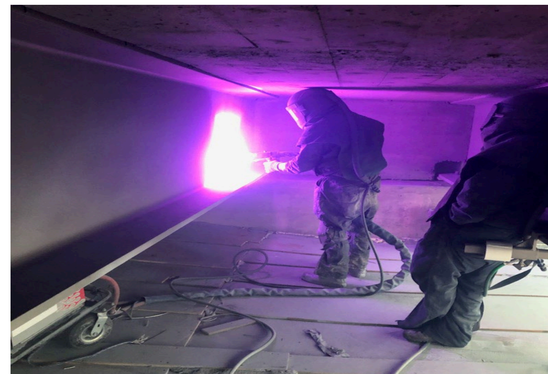
Application of Metalizing
