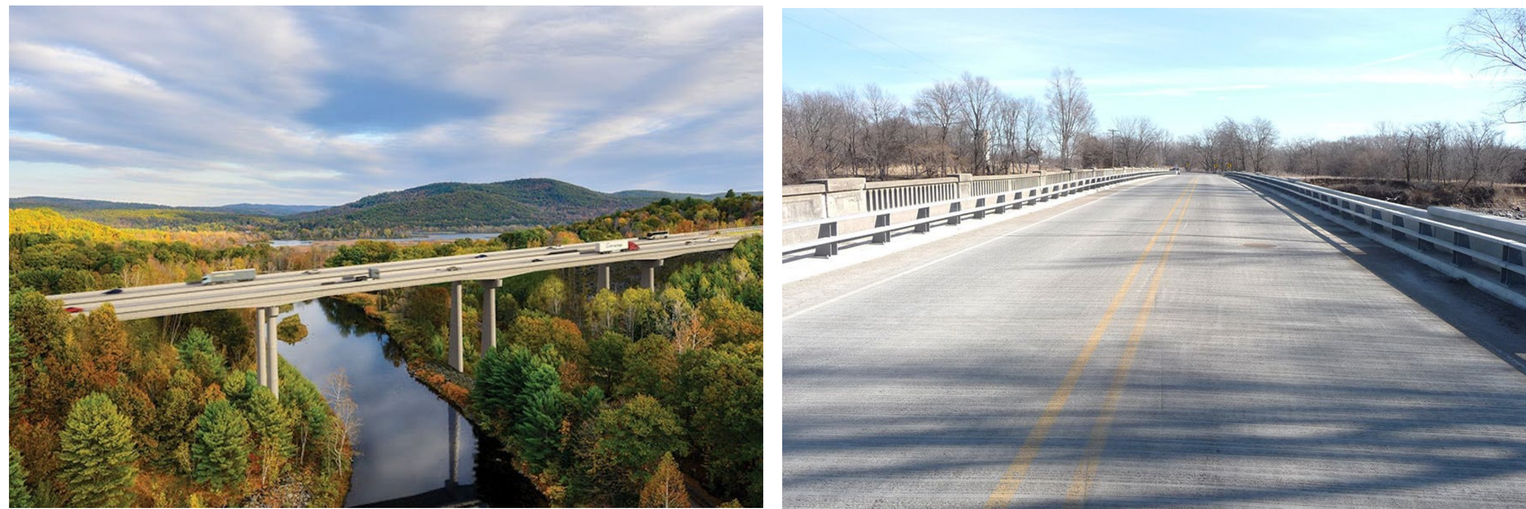
Figure 1. Typical images of a bridge and a bridge deck
