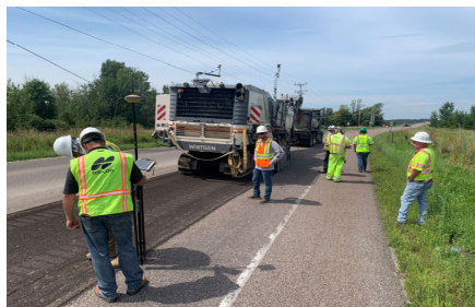
Figure (Left): Spot checking mill cut depth
