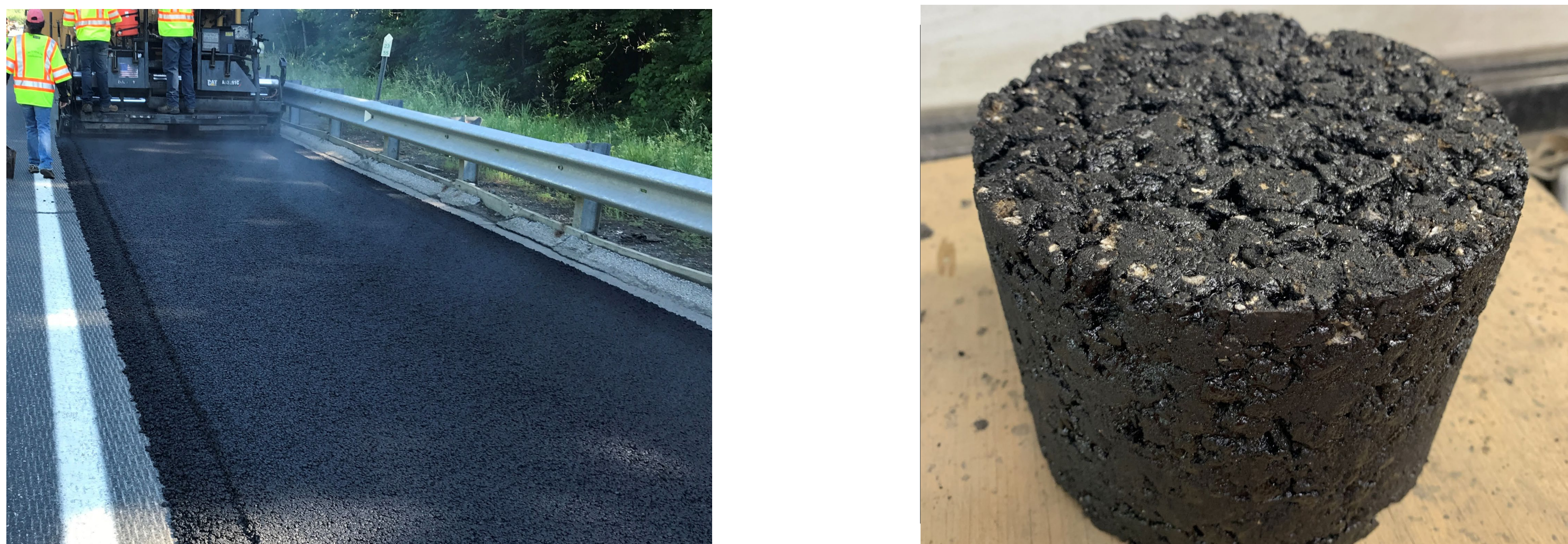
Figure 2. SMA construction, and an SMA sample for acceptance testing
