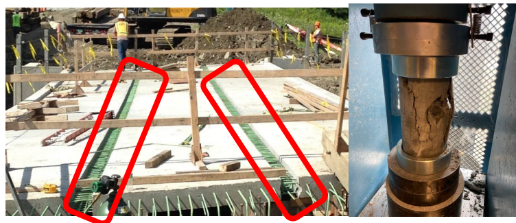
Left: VTrans ABC Connections (in red boxes) ready for RSC placement
