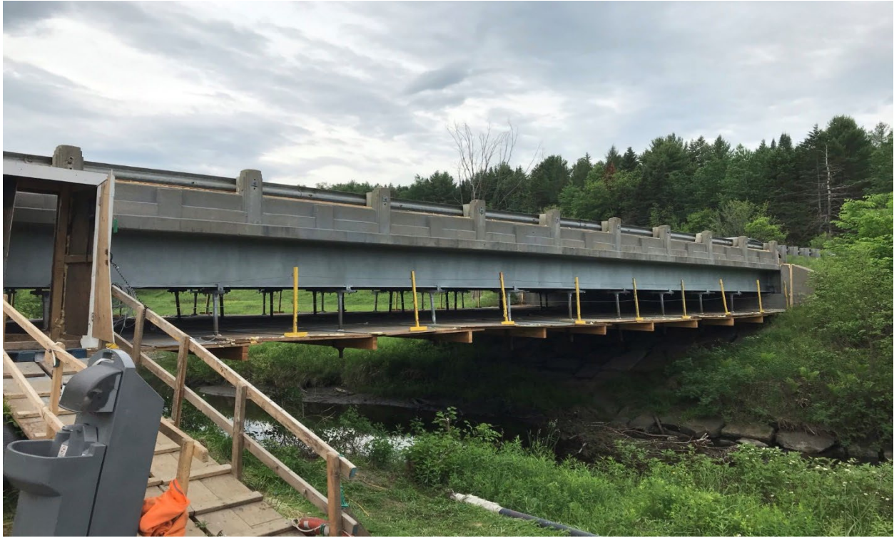
Work Platform Suspended from Beams
