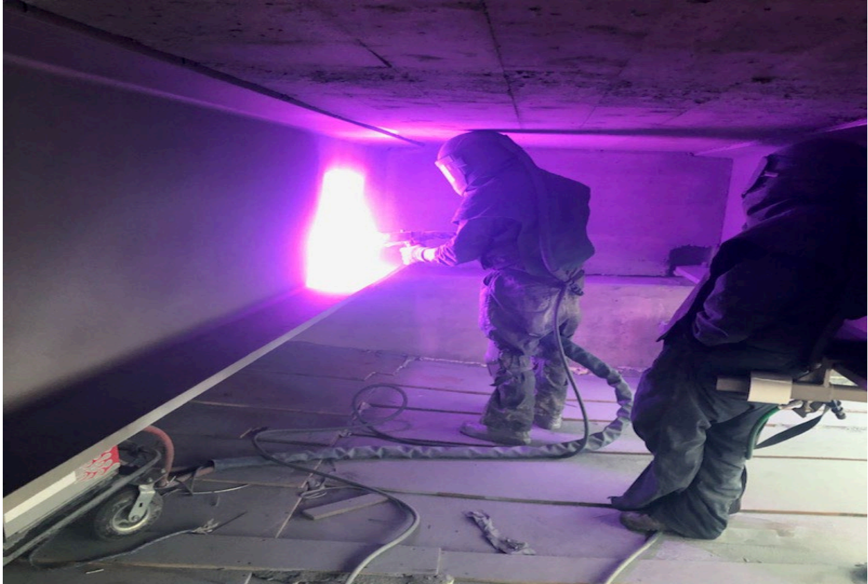
Metalizing Inside the Enclosure
