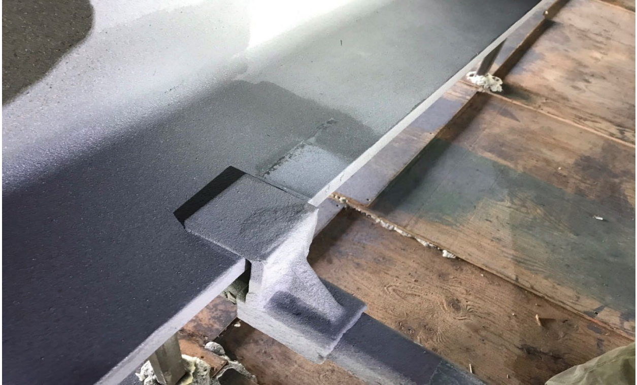
Repair Areas for Hanger Attachment
