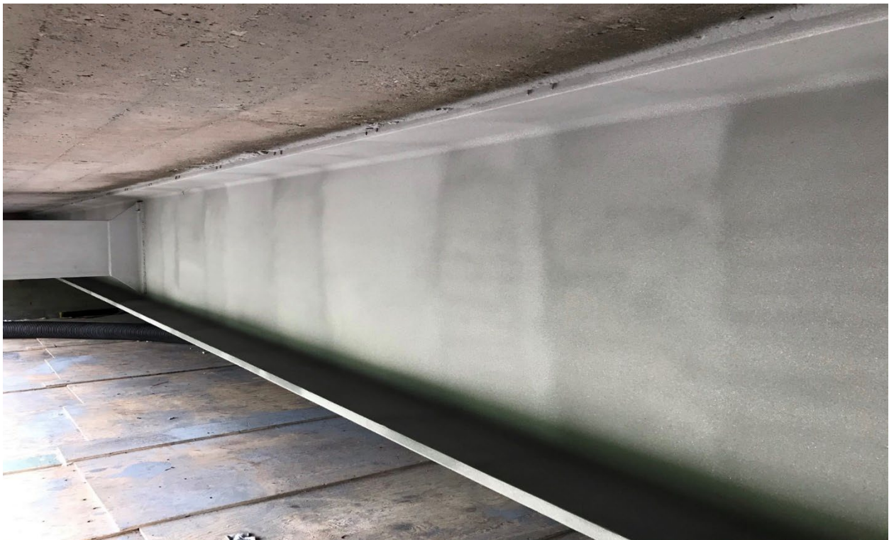
Streaks in the Final Coating
