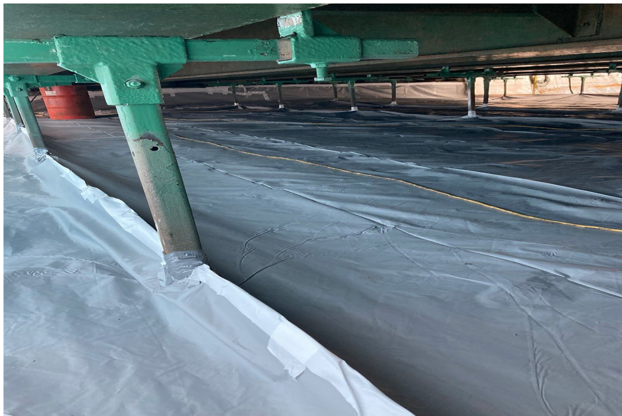
Bottom of Sealed Work Platform
