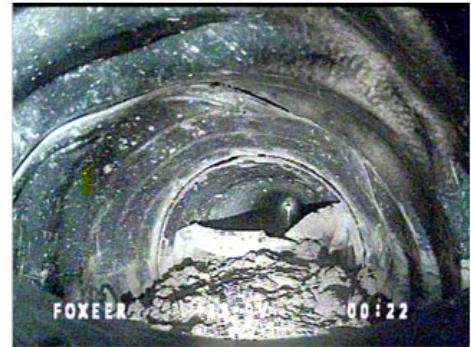
Fig. 2 Distressed culvert
