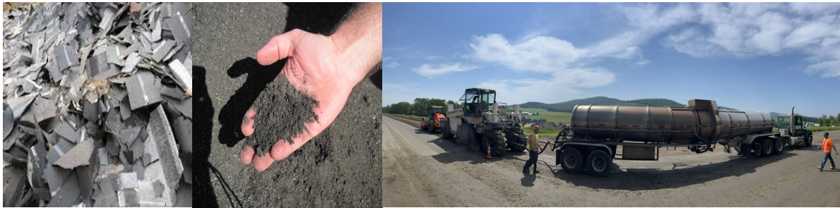
From left: “As is” architectural waste shingles; resized processed waste shingles; first pass reclamation from VTrans Marshfield-Danville project (reclaimer and water tanker)
