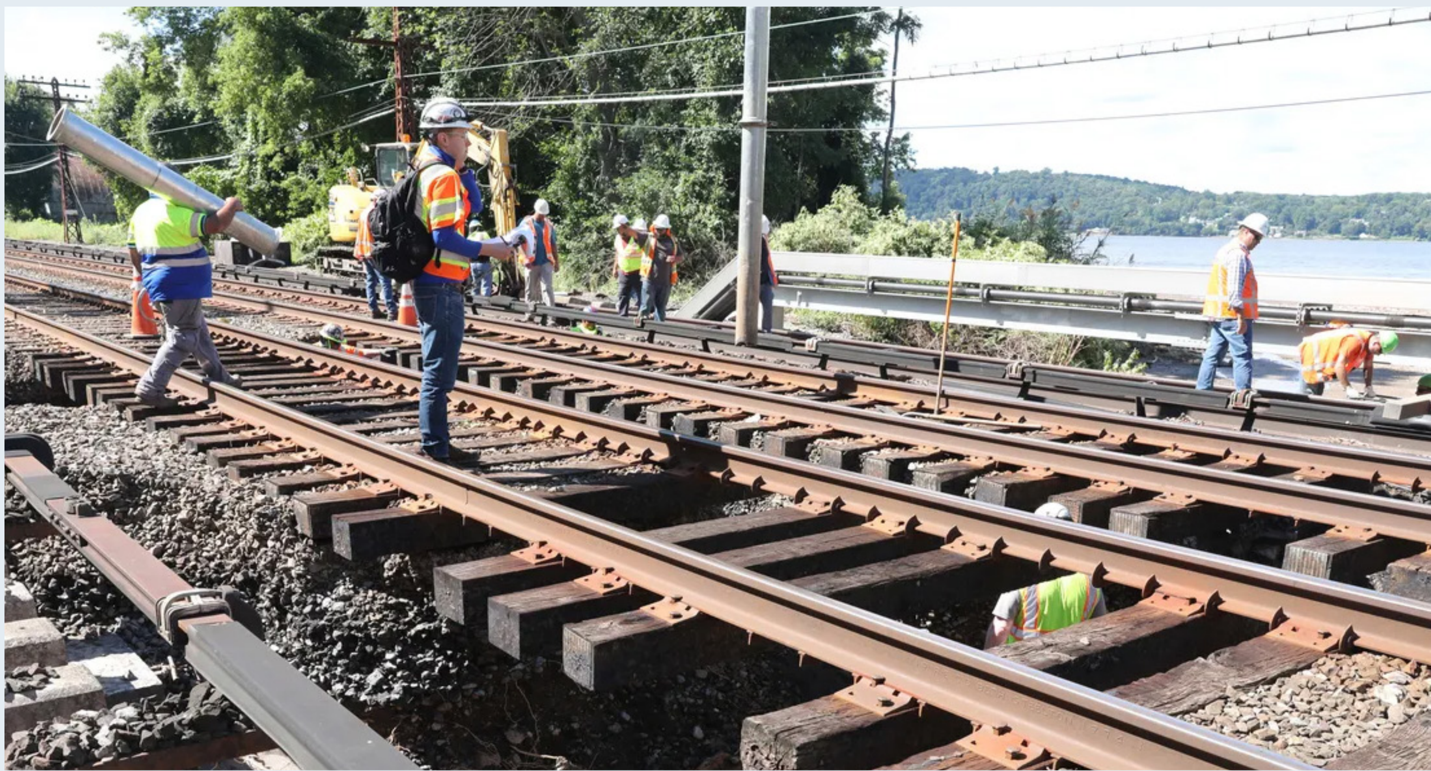
Bridge Washout after Hurricane Ida
