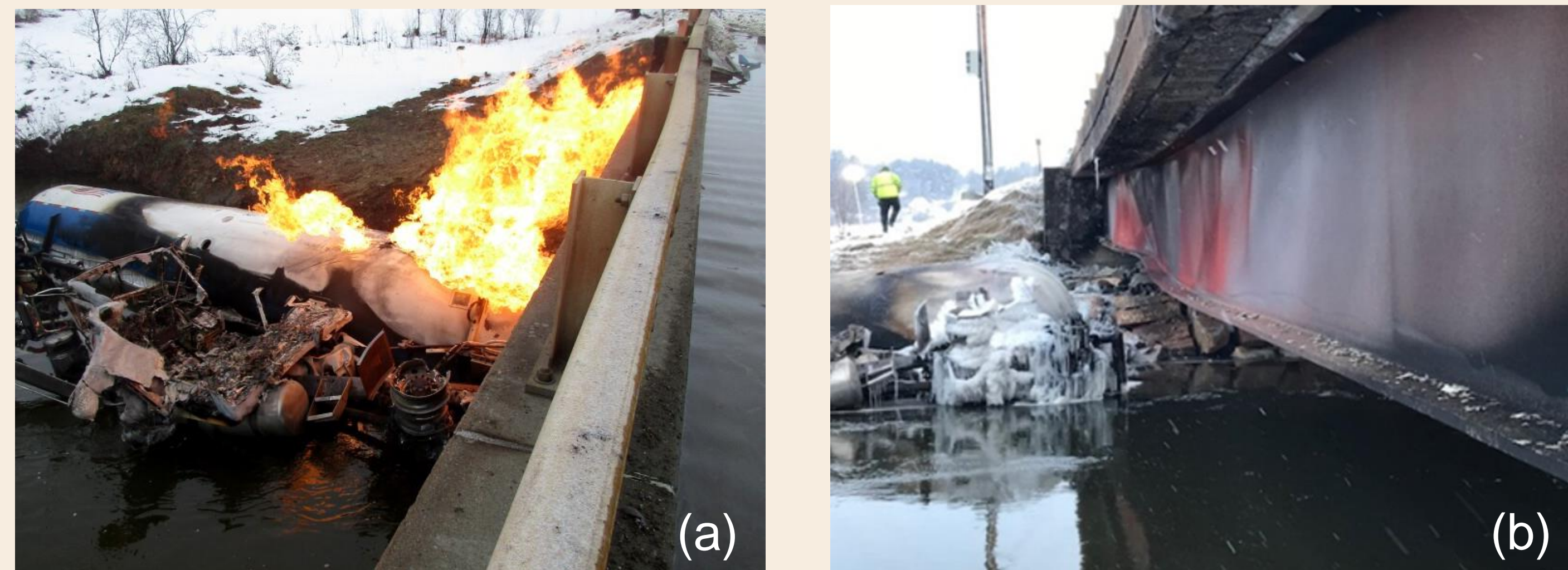
Figure 1. Photos of (a) Bridge VT 129 during fire, and (b) after fire extinguishing.
