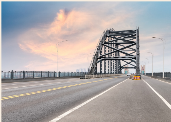
Figure 1. Typical Bridge Deck
