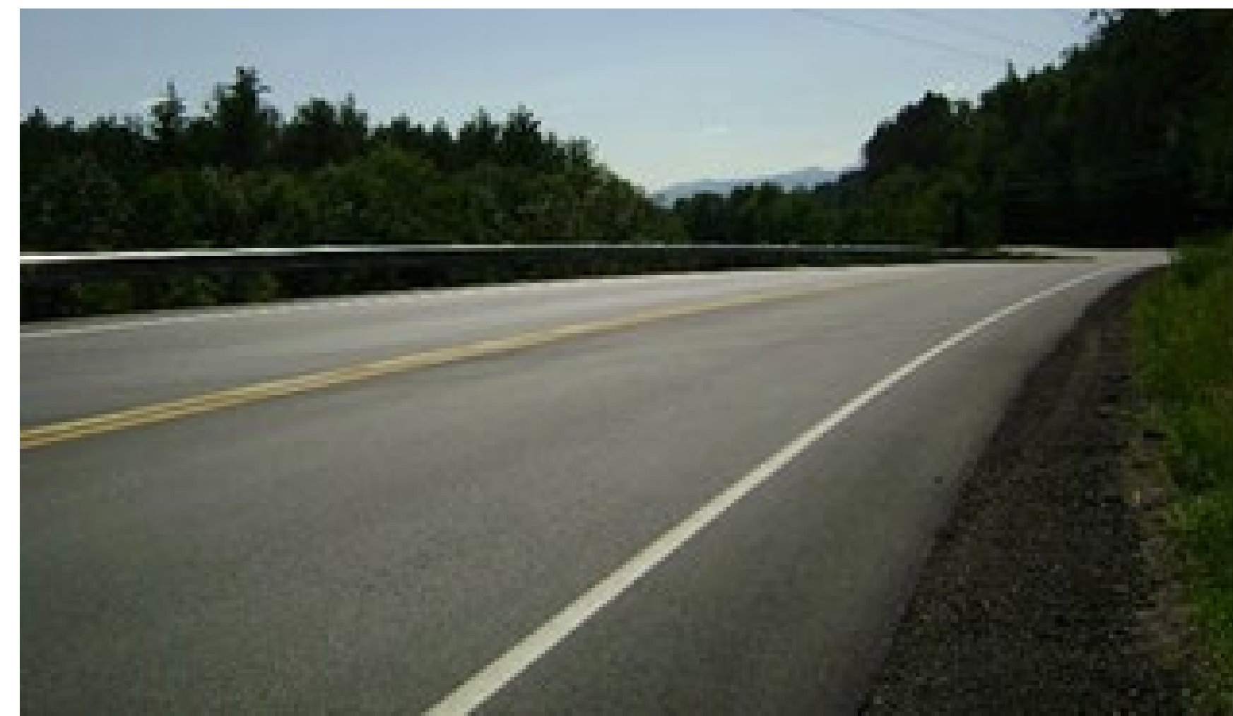
Figure 1. New pavement in Wolcott, VT.
