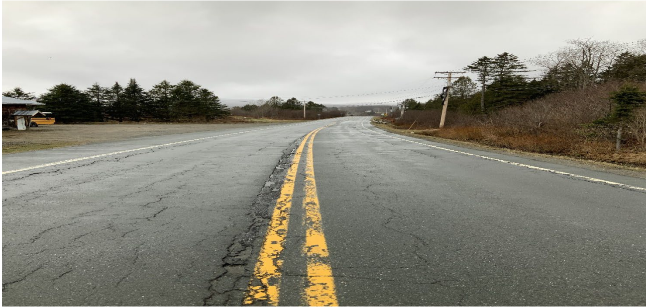
Norton MM 5.80: Pre-placement Conditions. Minimal rutting & extensive cracking
