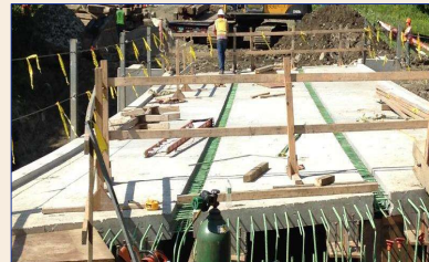
Figure 1. Accelerated Bridge Construction with Field Placed RSC Connections.
