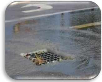
Photo: Road stormwater collection
