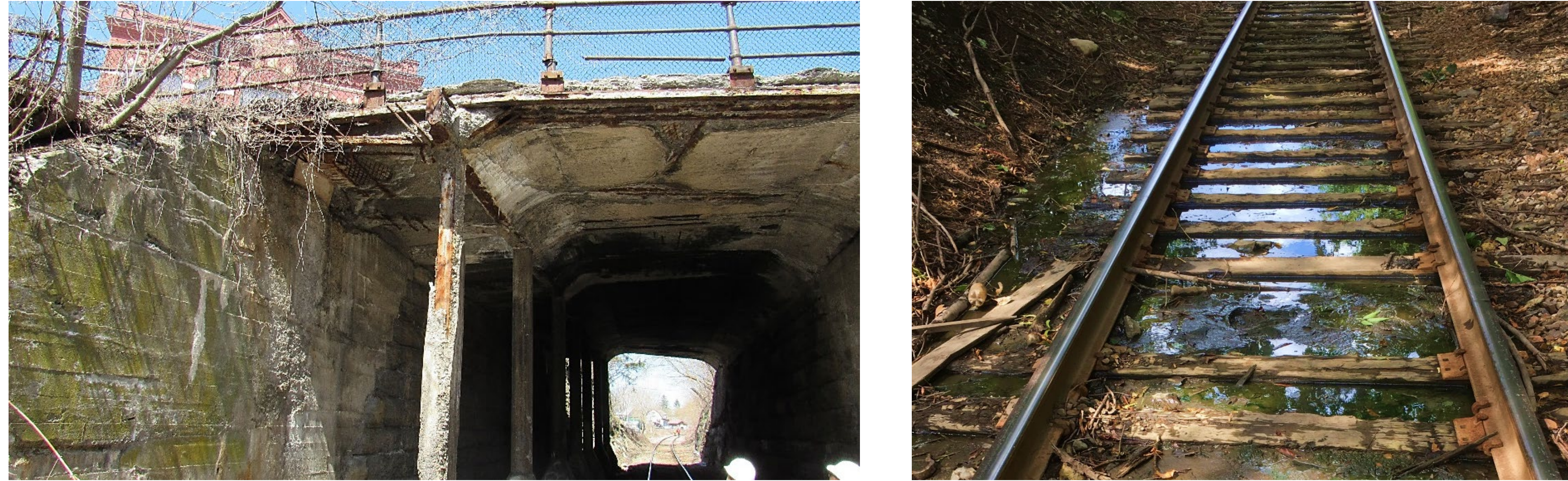
Figures: Old Bridge Deterioration, Pour Drainage of Old Rail
