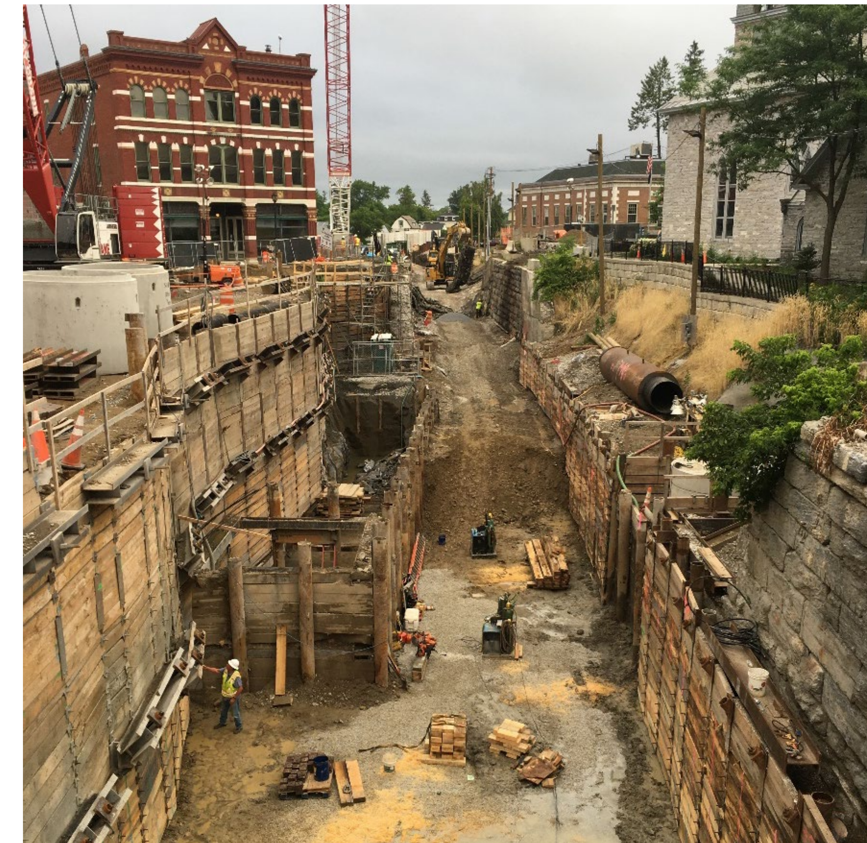
Figure Tunnel excavation
