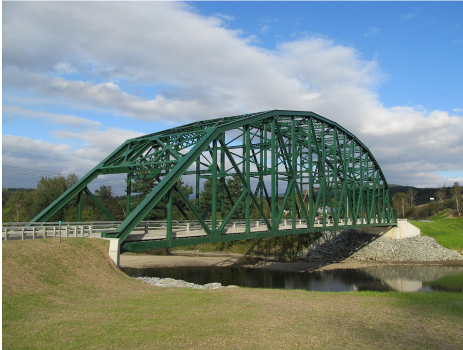
Checkered House Bridge Richmond VT
