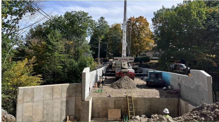
Construction and Maintenance
