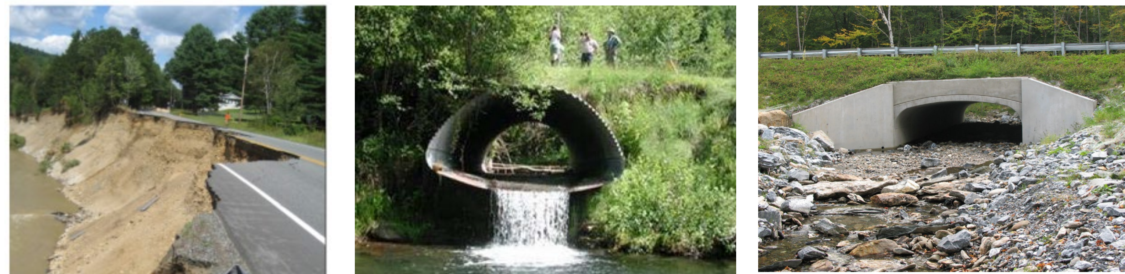
Figure 1. RHGCs (at right) are used to predict width, depth, and cross sectional area of the bankfull discharge (R.I. of Q1.5), to support flood-resilient sizing of infrastructure and permit passage of aquatic organisms (above).
