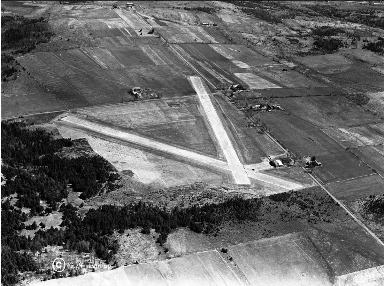
FIGURE 23: Aerial View of Barre-Montpelier Airport, 1939 (Landscape Change 1939)
