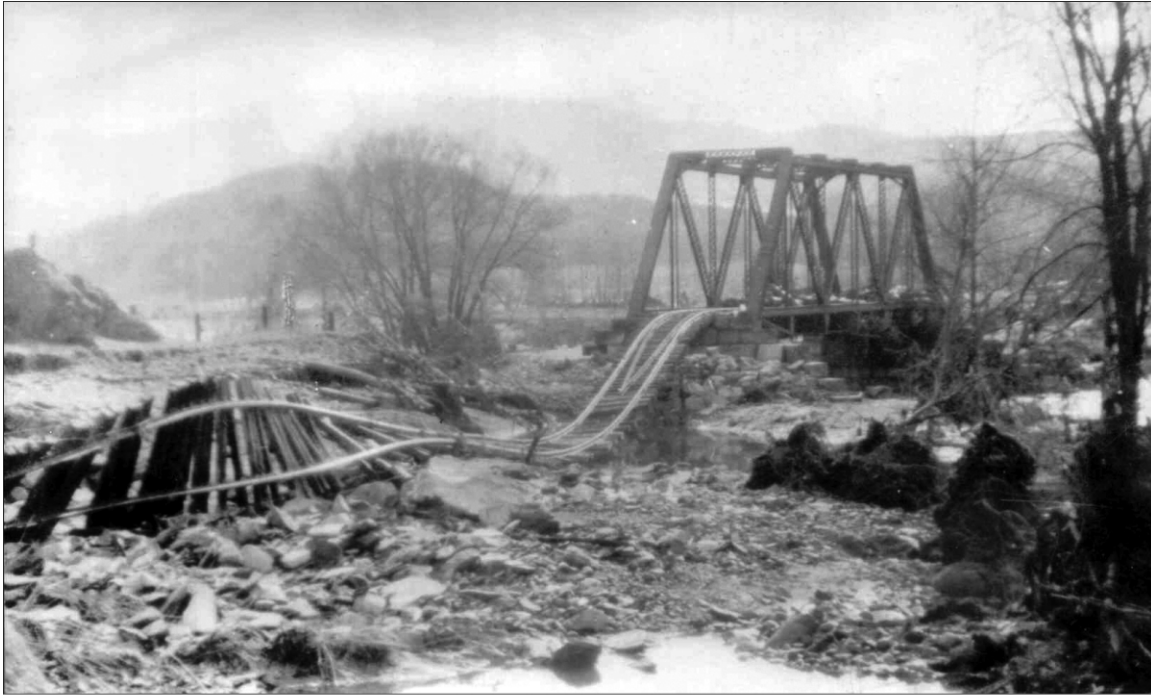
FIGURE 20: Damage to Railroad After Flood of 1927 (Landscape Change 1927)
