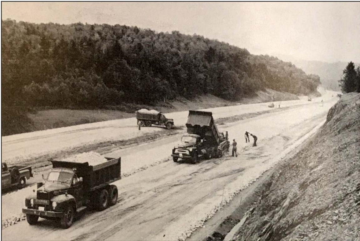
FIGURE 12: Constructing the Base on Vermont's First Interstate Highway Link (Vermont State Highway Board 1956-1958)
