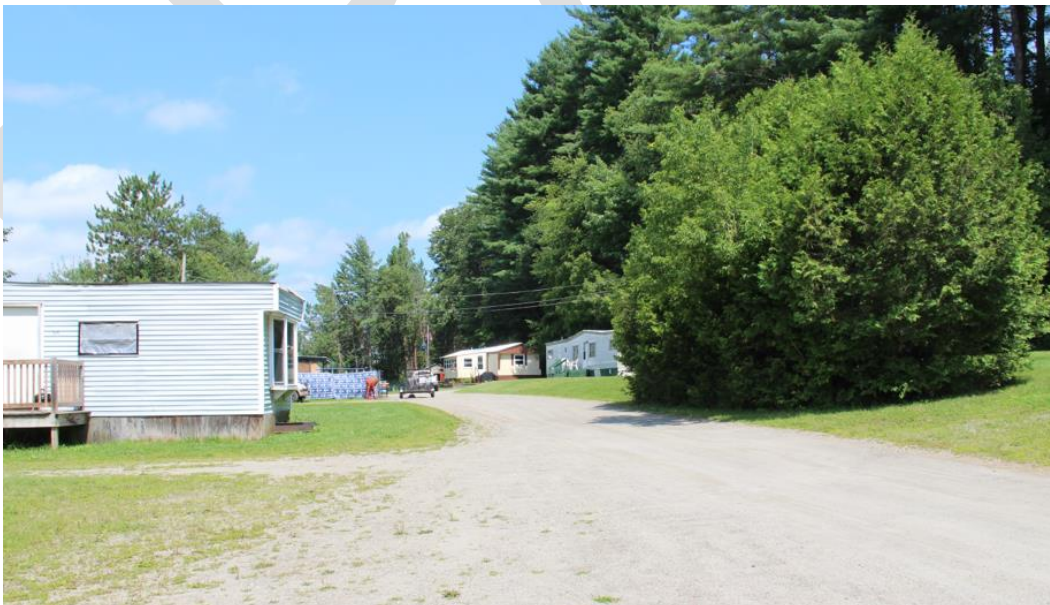
Figure 52. The McGill Avenue park. Units are arranged perpendicular and parallel to the drive on either side to maximize the number contained within the park.
