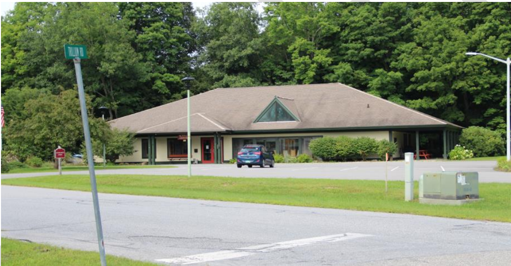
Figure 43. The community center at Williston Woods.
