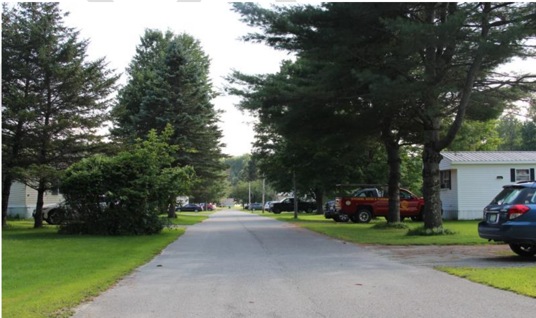
Figure 37. View of the Tucker Mobile Home Park including streetlights, driveways, and landscaping.
