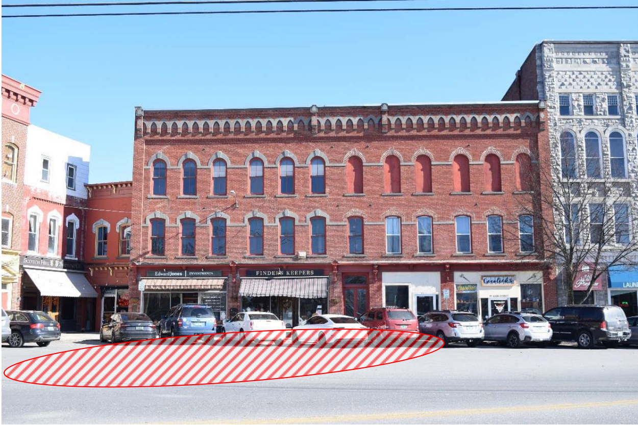
Figure 11. Approximate location of pedestrian plaza.
