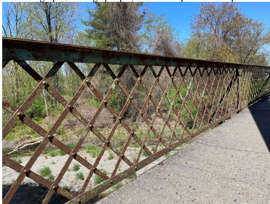
Photograph 6: Bridge pedestrian railing. Map ID 1.
