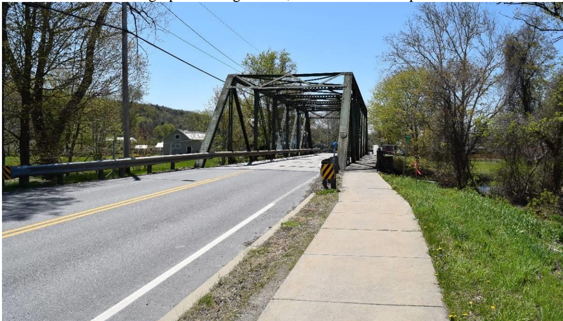
Photograph 2: Bridge 4 looking south. Map ID 1.
