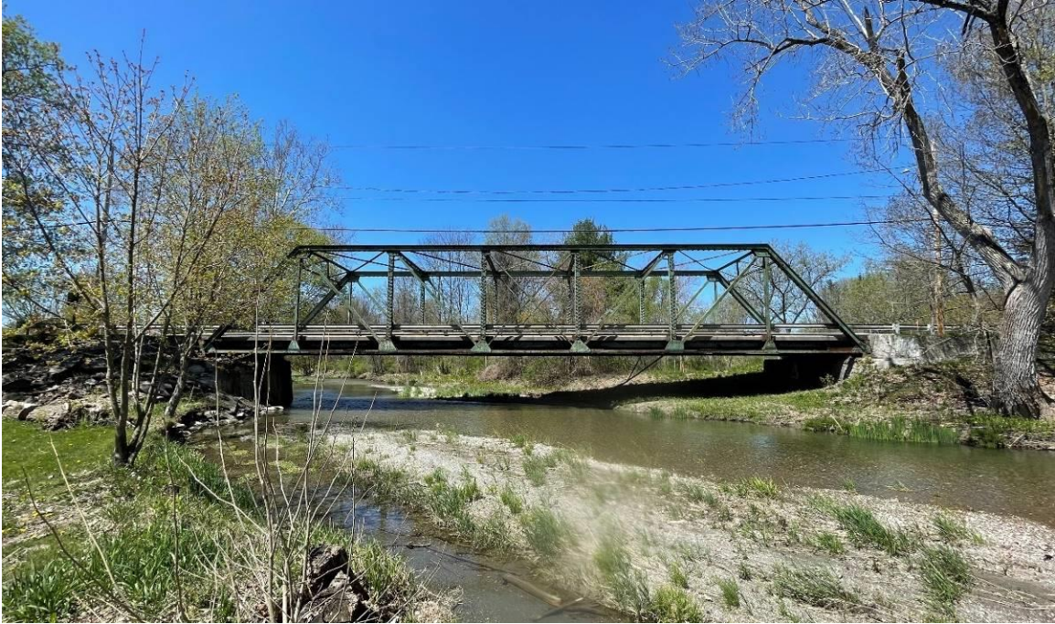
Photograph 1: Bridge No. 4, east elevation. Map ID 1.
