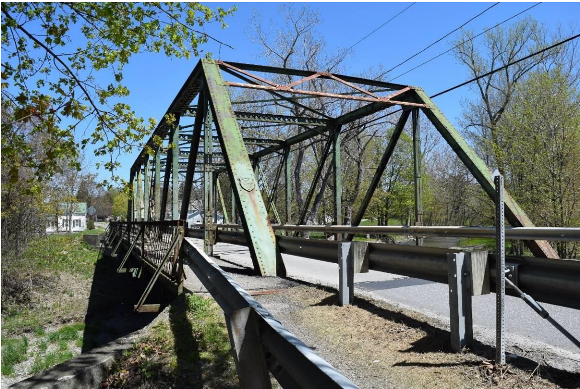
Photograph 3: Bridge No. 4, southwest quadrant, looking northeast. Map ID 1.
