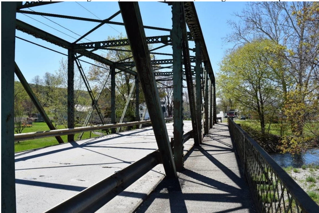
Photograph 4: Bridge No. 4, looking south. Map ID 1.
