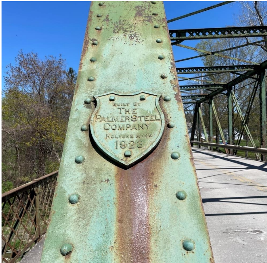
Photograph 5: Bridge plaque, southwest quadrant. Map ID 1.
