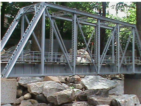
Pratt Through Truss
