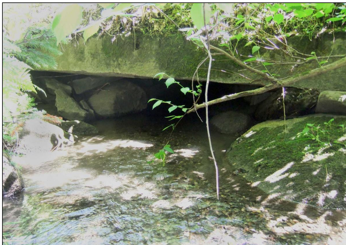
FIGURE 6: This box culvert of split and cut granite quarry stone on Sterling Hill Road in Barre Town (WA-BAT-001) is the longest span culvert surveyed with an opening 84" wide and 24" high.
