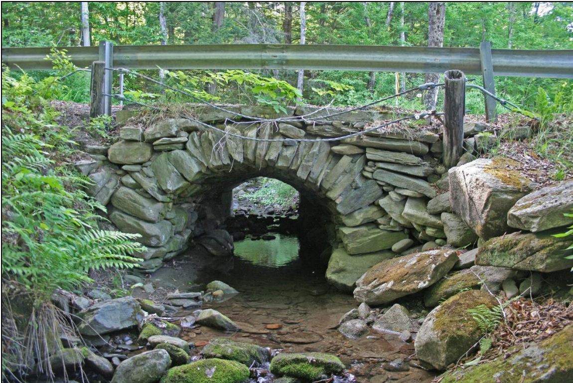
FIGURE 13: Stone arch culvert on Hill Road, Brookline (WI-BRO-001). This is the one stone arch culvert inventoried by the Vermont culvert survey. It is a segmental arch with a span of 80 inches. It is built entirely of fieldstone including the arch which includes a few naturally wedge-shaped stones, flat stones and shims to establish good contact (bearing) between the primary arch stones. The upstream end of the culvert was lengthened about 12 feet with the addition of a concrete arch, visible above in silhouette thru the opening and also in Figure 16 below.
