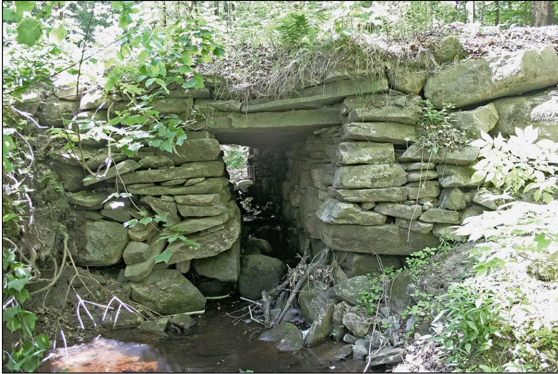
FIGURE 8: Wiswall Hill Road, Newfane (WI-NEW-003). This rubble and fieldstone box culvert consists mostly of flat rubble stone with no evidence of splitting. The stone was evidently gathered from an outcrop that had naturally broken up along its thin bedding planes – a desirable source of wall stone. The dry-laid masonry utilizes stones of all shapes and sizes and small chinking stones to achieve a tight and stable wall. But the use of large round fieldstone boulders at the base (at lower left) that are more easily displaced than flat stone, was a poor decision.
