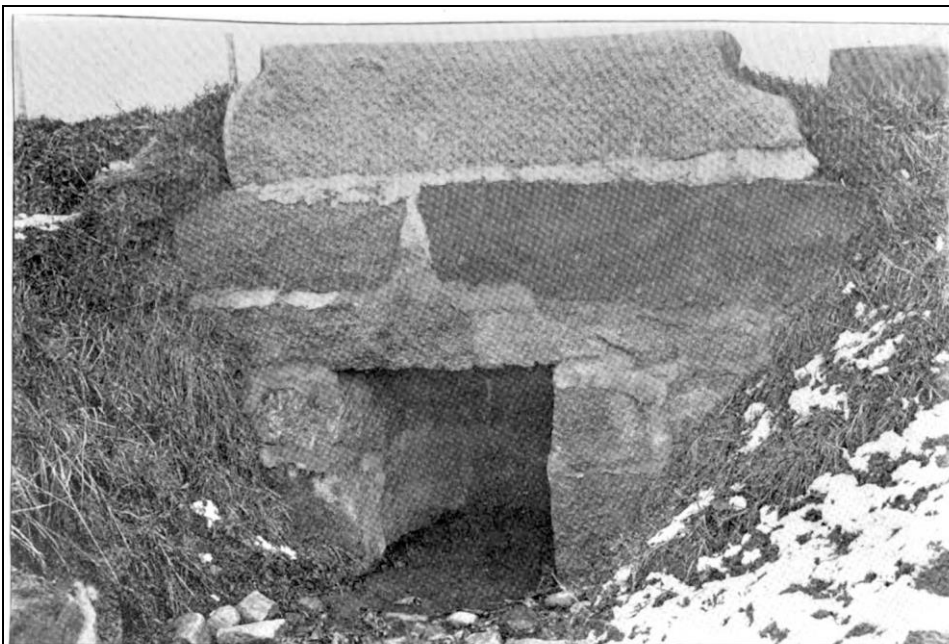
Cut No. 15—Stone culvert built in Glover in 1905.
