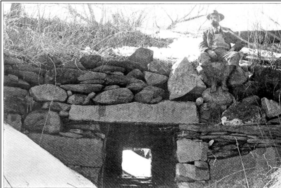
Cut No. 14—Stone culvert built in East Montpelier in 1897. 3\frac{1}{2} \times 3\frac{1}{2} \times 30 with 18 foot fill.
