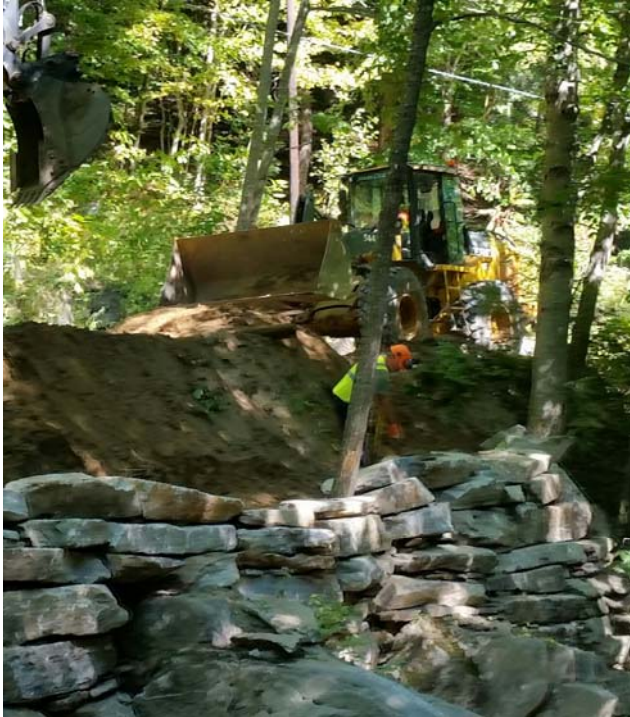
Installation of a Better Roads grant project in Chester, VT
