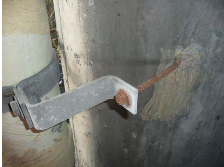
Figure 2 - Deformed Bolt
