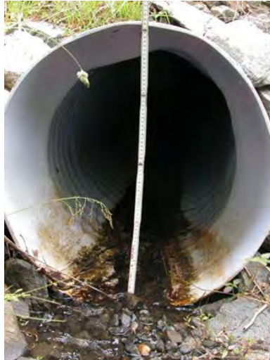
Figure 3: Inlet of 24-inch pipe, 2007
