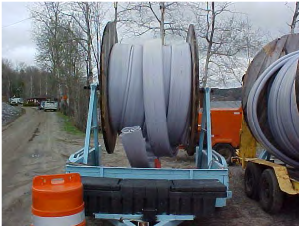
Figure 1 Spooled Ultraliner on the project site.
