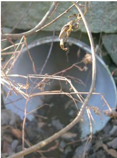
Figure 5: 18-inch pipe outlet, 2004
