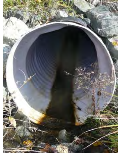
Figure 4: Inlet of 24-inch pipe, 2010
