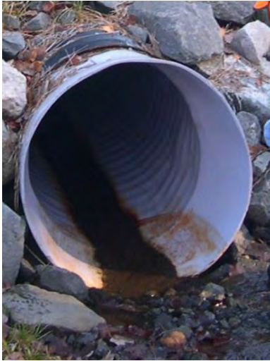
Figure 2: Inlet of 24-inch pipe, 2004
