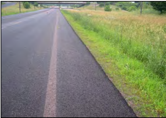
Figure 2- Recess for Yellow Edge Line
