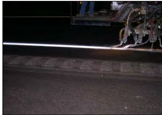
Figure 4- White Edge Line Application
