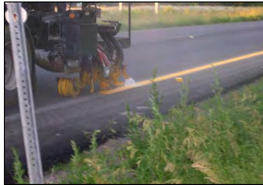
Figure 3-Yellow Edge Line Application
