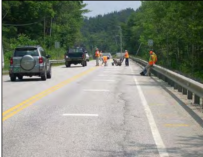
Figure 1: Installation – Bondville headed southbound
