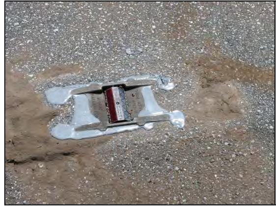
Figure 2 – Hallen Marker with Epoxy
