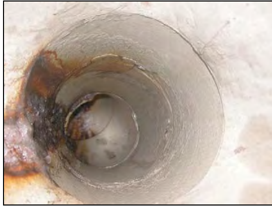
Figure 5 – Iron-Oxide Discoloration
