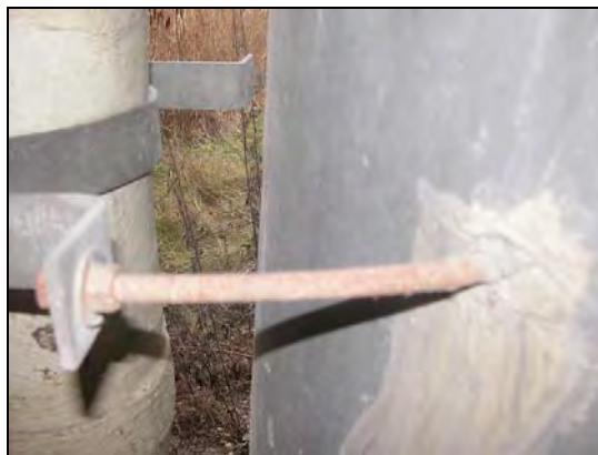
Figure 4 – Bolt Deformation
