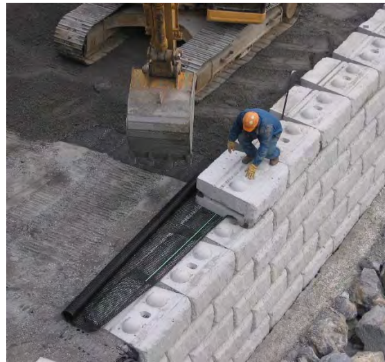
Figure 6: Geogrid installation
