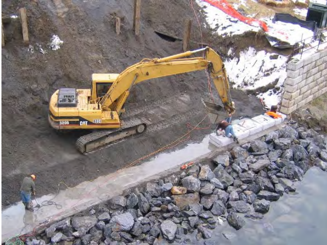
Figure 5: Installation of 1 st row of blocks
