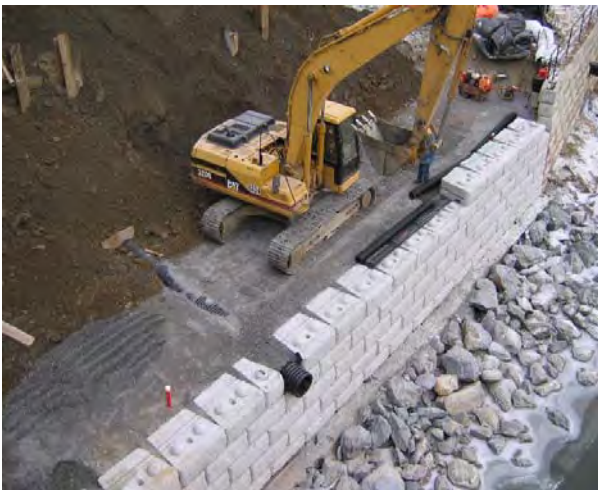
Figure 7: Drainage pipe installed through Redi-Rock™ wall.
