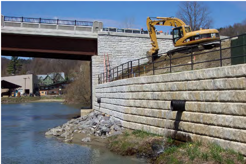
Figure 9b: Completed Redi-Rock Retaining Wall
