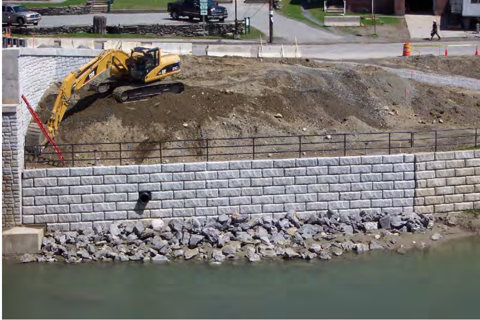
Figure 9a: Completed Redi-Rock Retaining Wall
