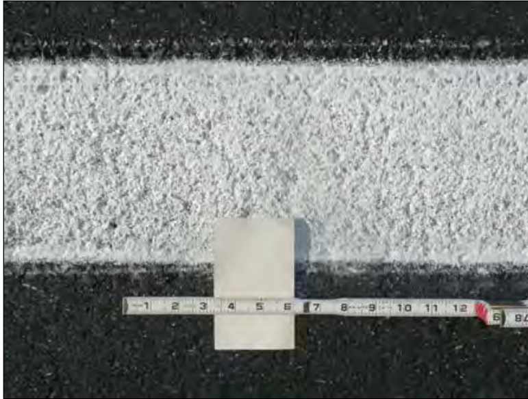
Figure 4. Appearance of the 3M LPM 1200 polyurea five days post-installation.
