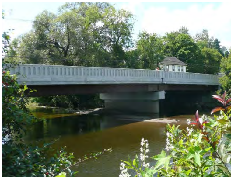
Figure 5. Overview of the Lyndon bridge.
