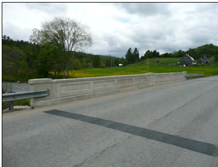
Figure 4. Overview of the Corinth bridge.
