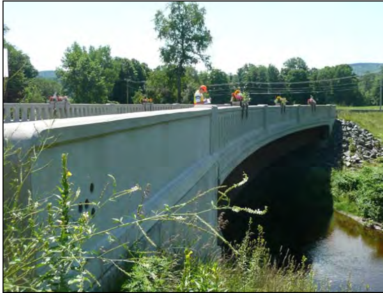
Figure 2. Overview of the Chester bridge.
