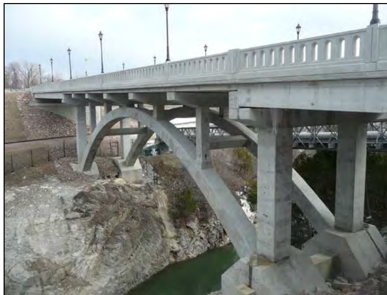
Figure 3. Overview of the Colchester - South Burlington bridge.
