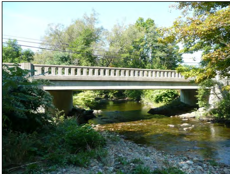
Figure 8. Overview of the Underhill bridge.
