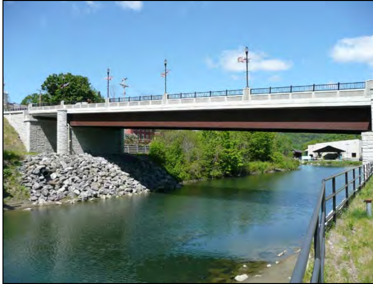
Figure 1. Overview of the Bethel bridge.
