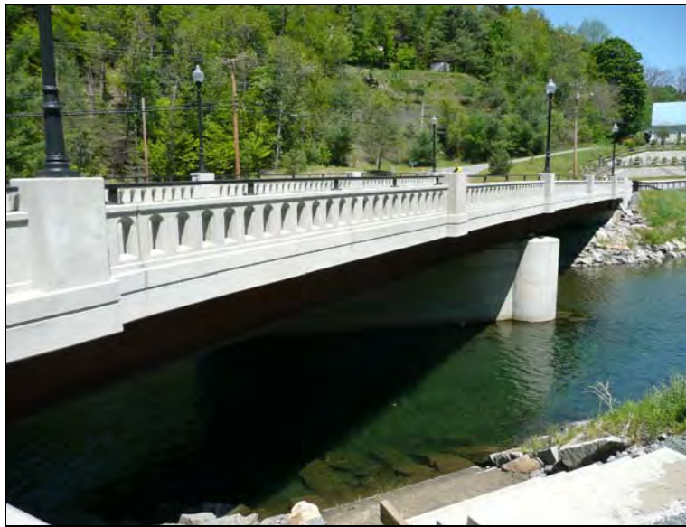
Figure 7. Overview of the Tunbridge bridge.
