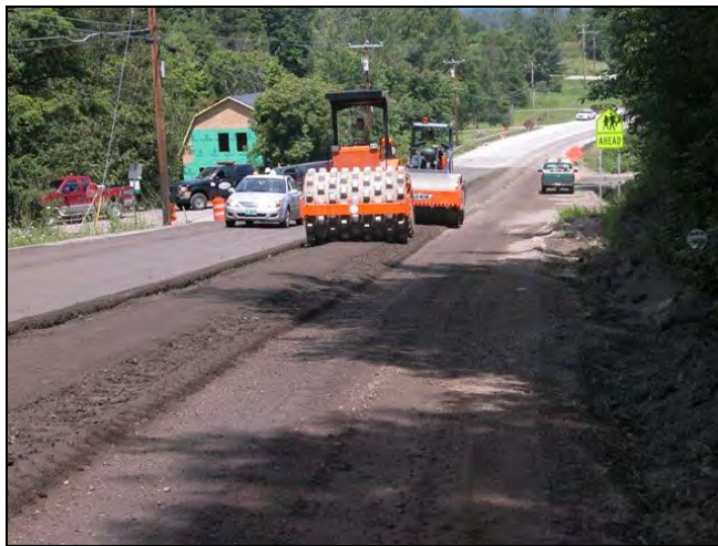
Figure 5 – Reclaimed Base Compaction
