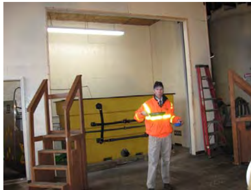
The Chimney Corners Salt Brine Manufacturing Facility
