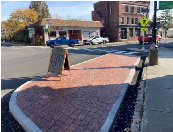
Figure 6: Permanent curb extension in Hardwick, VT
