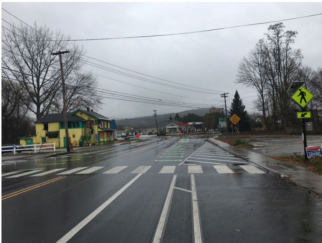
Figure 3: Bicycle lane, crosswalks, and lane restriction in West Rutland, VT. Photo by Matt Bogaczyk
