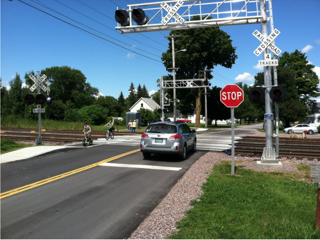
Figure 4: Railroad crossing in St. Albans, VT.
