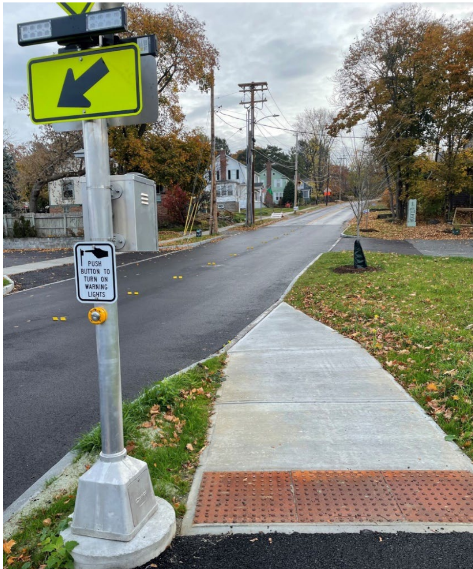
Figure 88: Bicycle ramp on Burlington HES 5000(18) roundabout
