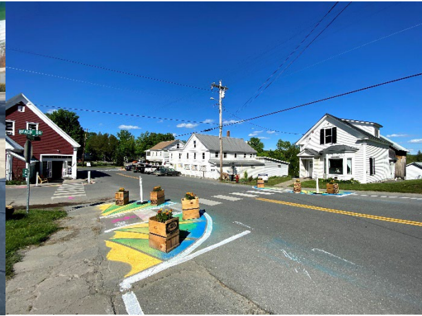
Figure 77: Temporary curb extension, photo by Local Motion
